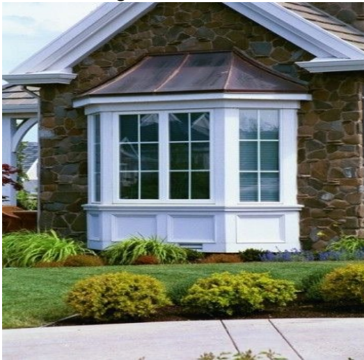
Photo showing location of work
